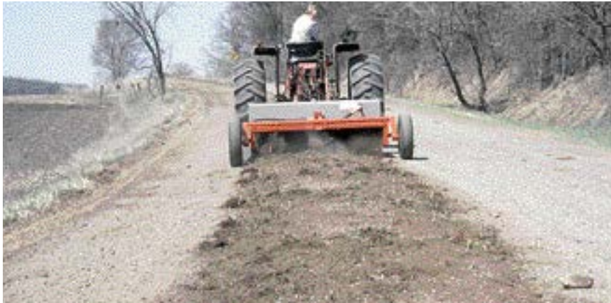
A machine made in Canada pulverizes gravel windrows into usable material on the roadway.
