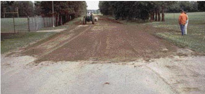
Another washboard-prone area is at the transition from paved to gravel sections as shown in this photo.
