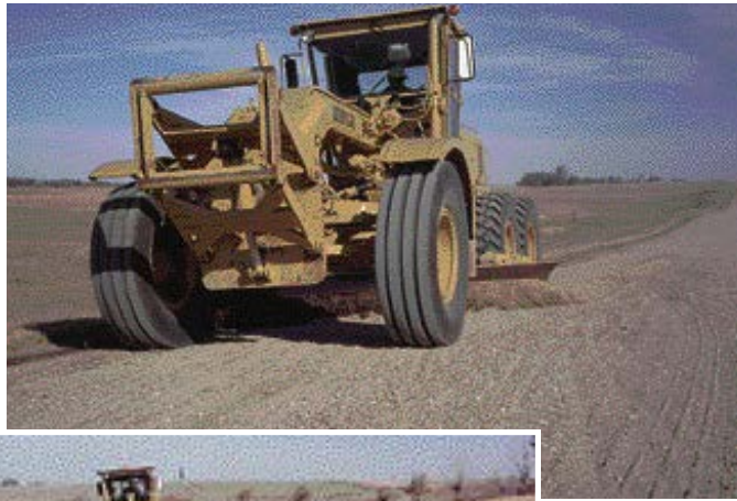
The existing surface gravel is cut loose and windrowed to the opposite side of the road.
