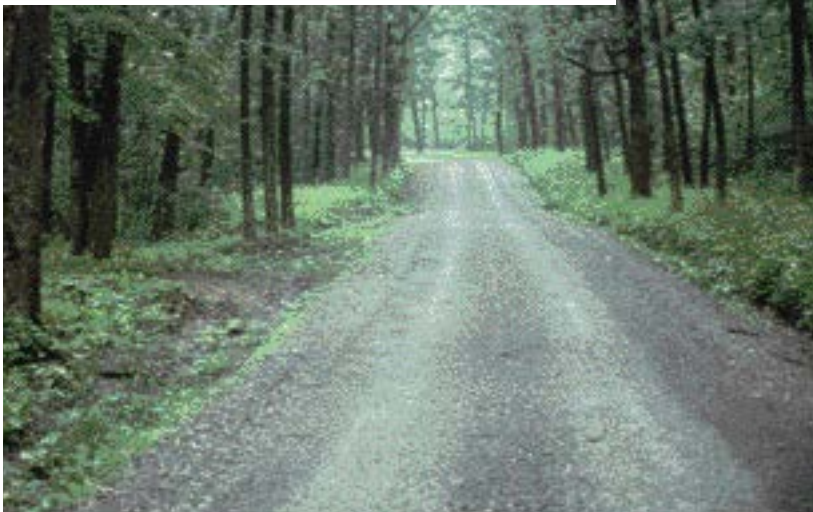
The road now performs very well after the stabilization was completed.
