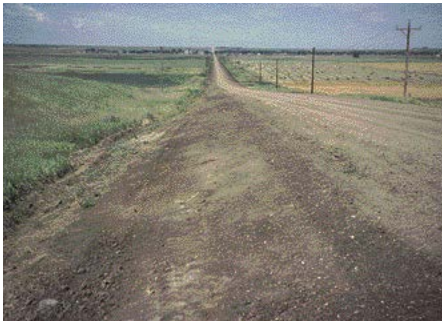
An example of a well shaped gravel road shoulder that slopes away from the driving surface and drains water to the inslope and ditch.
