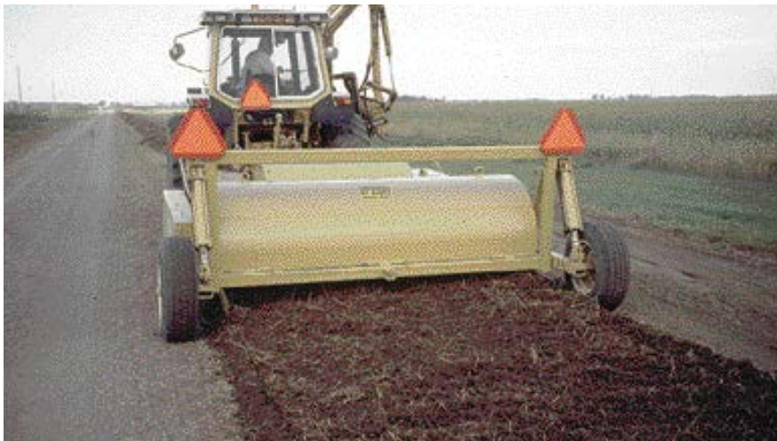
A machine fabricated specially by Hyde County in South Dakota to pulverize heavy windrows of recovered gravel and grass from the shoulder. It quickly breaks down windrows for reuse on the road.
