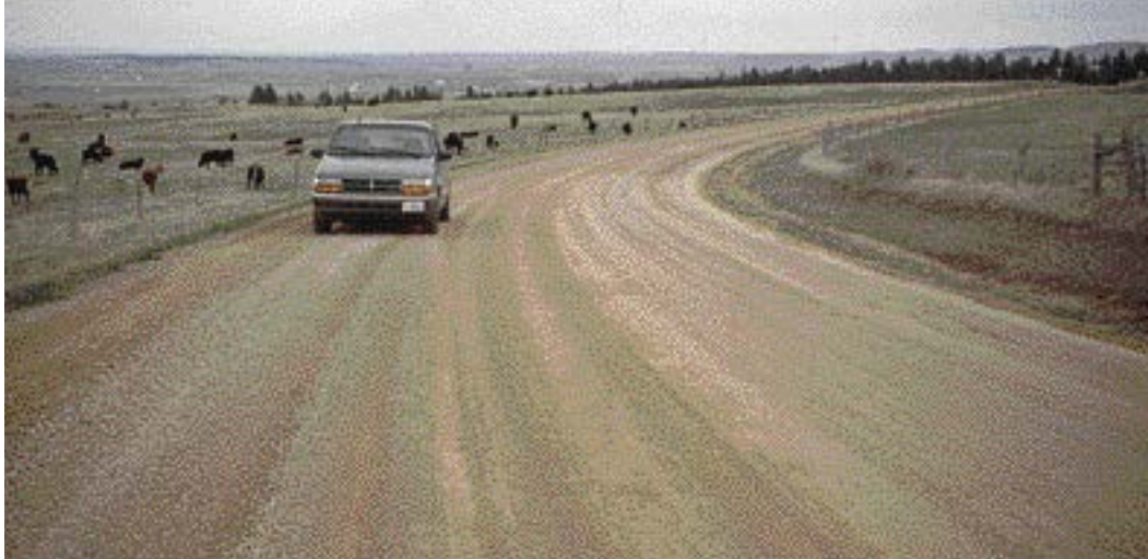
This superelevated road section makes driving safer.
