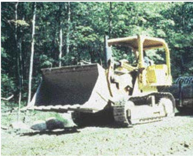
The crawler/loader was used to spread the material over the fabric and is now being used to pull a grid roller to smooth the surface.
