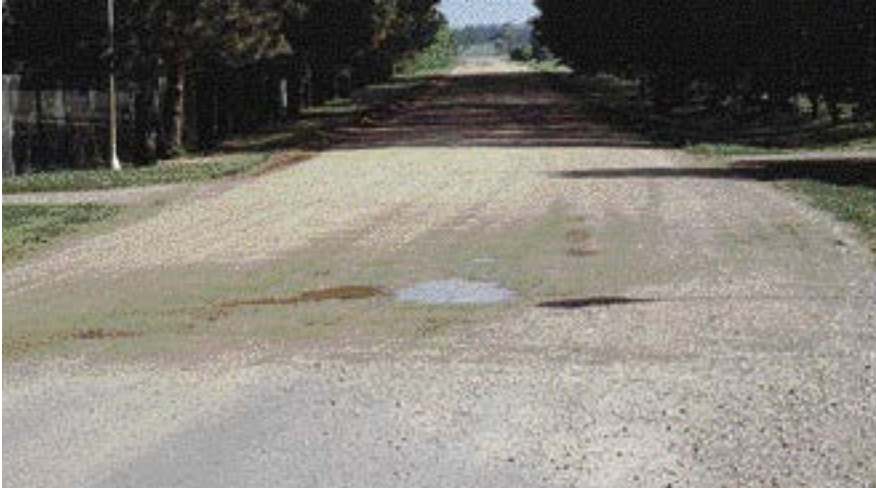
It is a good practice to loosen, mix, reshape gravel in a washboard-prone area while it is moist.
