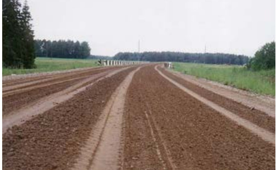
Example of a good blend of material for gravel surfacing. (Courtesy of Road Research Ministry of Roads/Transportation, Sweden)
