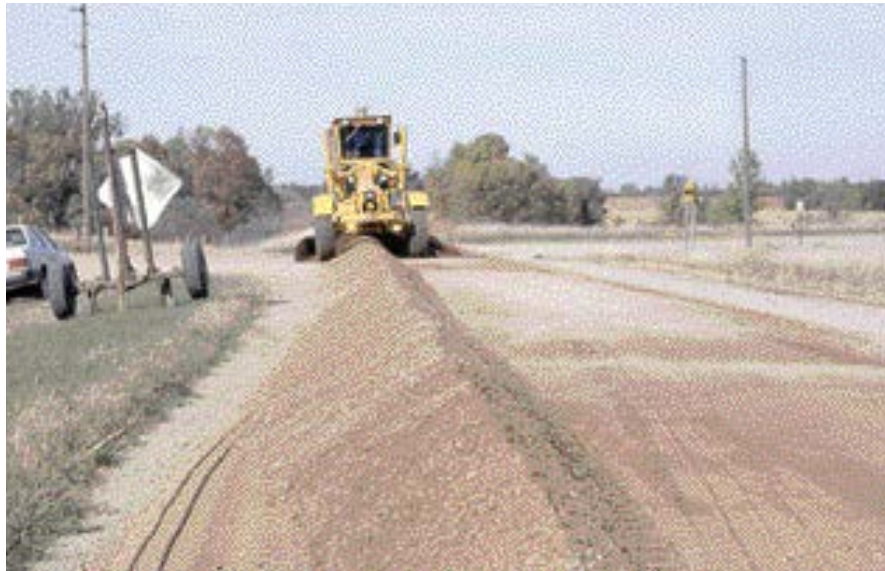
Only after completely windrowing and equalizing does the operator begin to place the material at a uniform depth across the roadway.
