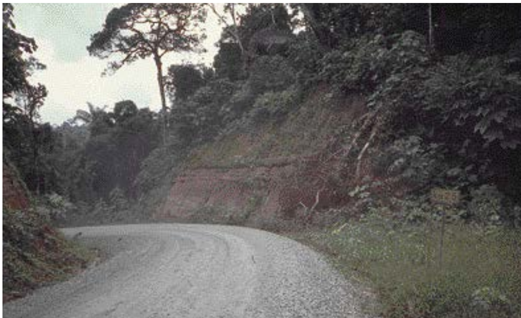
This road in Ecuador has excellent superelevation in the curve. It also has good shoulder drainage and ditches on both sides of the road. (Courtesy of Ron Anderson, Tensar Earth Technologies, Inc., USA)
